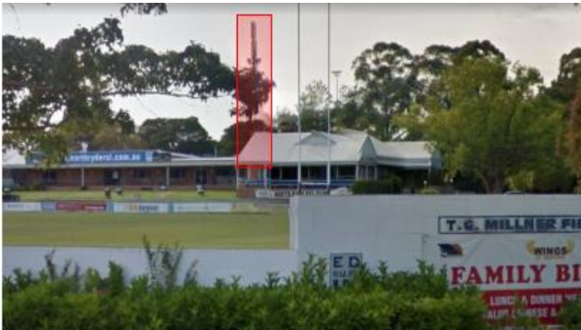
Mobile Carrier Base Station mounted on mast
